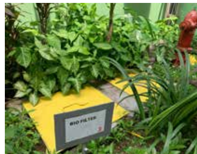
Bio Filter 3 : Biofilter sumber limbah dari gedung utama dan sumber limbah dari bekas air wudhu mushola. Bio Filter 3: Biofilter waste source from the main building and the source of waste from the former water ablution prayer room.
